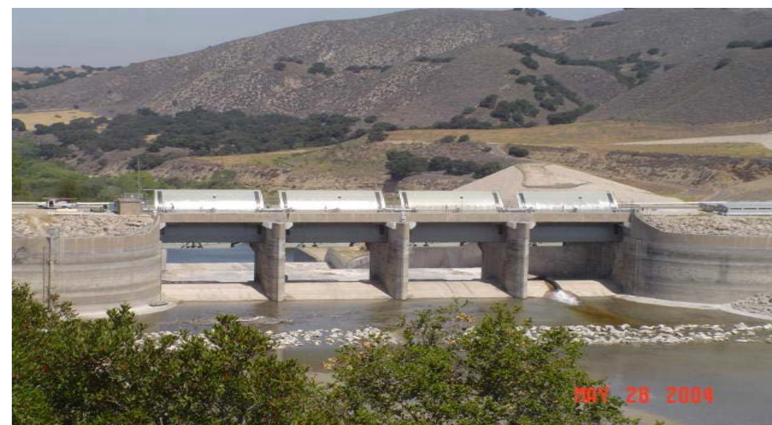
Bradbury Dam with all four radial gates open and the 4-foot flashboards on top
